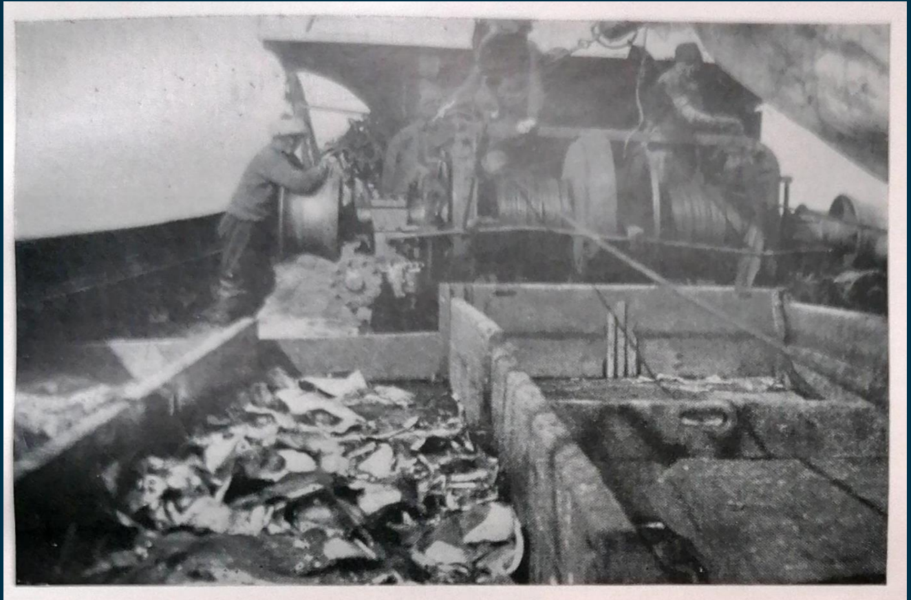
Steam-powered winch on board a fishing vessel. After Lübbert in Schnakenbeck 1953
